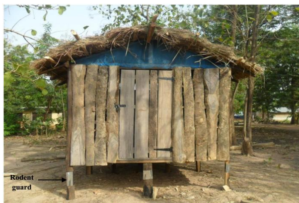
Fig9. The improved yam storage structure with rodent guards fixed
