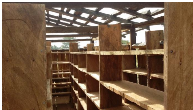
Fig7. Arrangement of shelves in the improved storage structure
