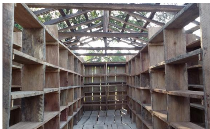
Fig4. Yam storage structure shelves constructed with Ceiba wood
