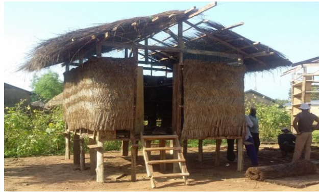
Fig5. An improved traditional yam storage structure with Zanna mat as covering material
