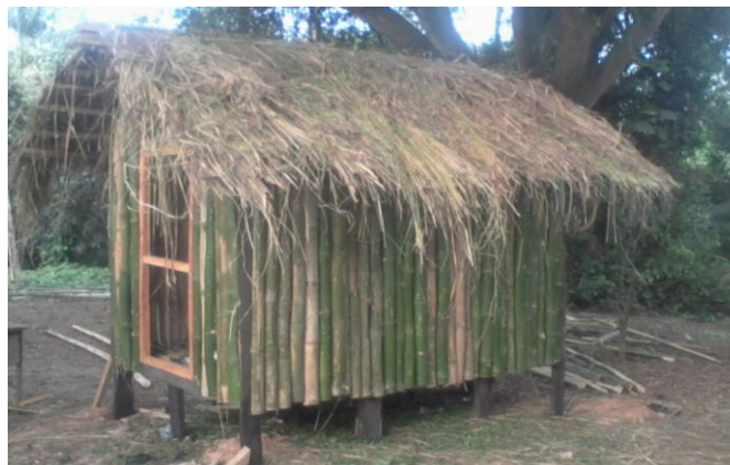
Fig3. Bamboo used as cladding and floor material for a yam storage barn
